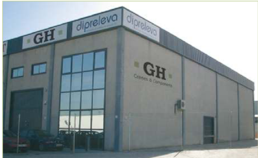
GH spare parts distribution center
